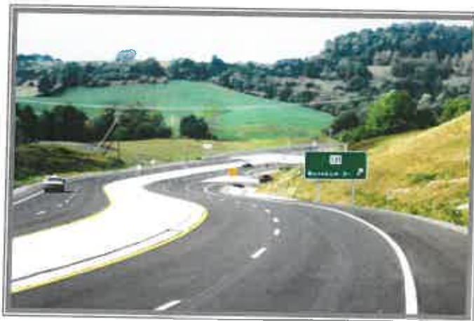
North Bridgeport Bypass
